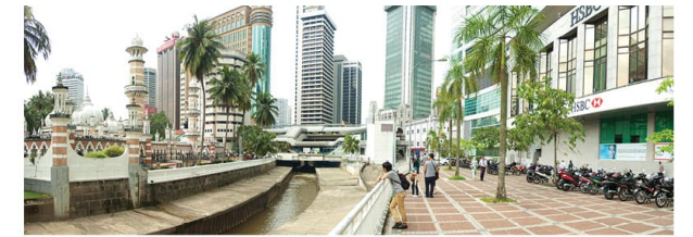
HSBC Walkway Before - Motorcycle parking and back alley
